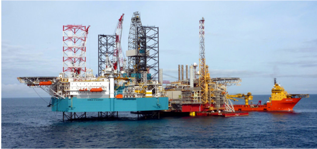
Production platform on the YME field
